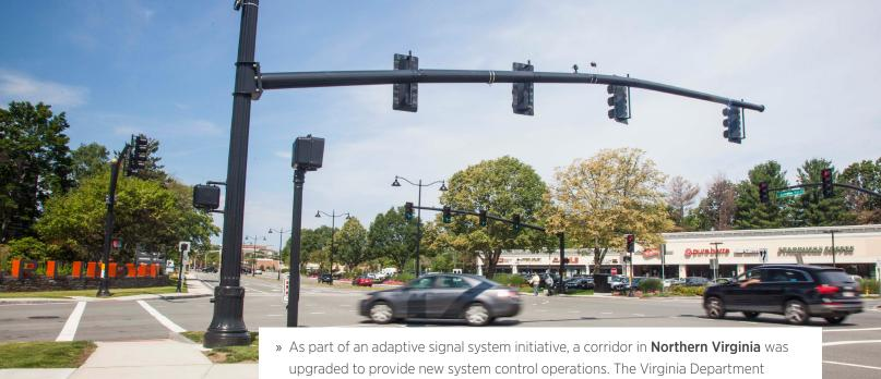
With the implementation of ASCT along the major arterials in Burlington, MA, traffic congestion is reduced, left-hand turns are more efficient, and progression is improved along the corridor.
