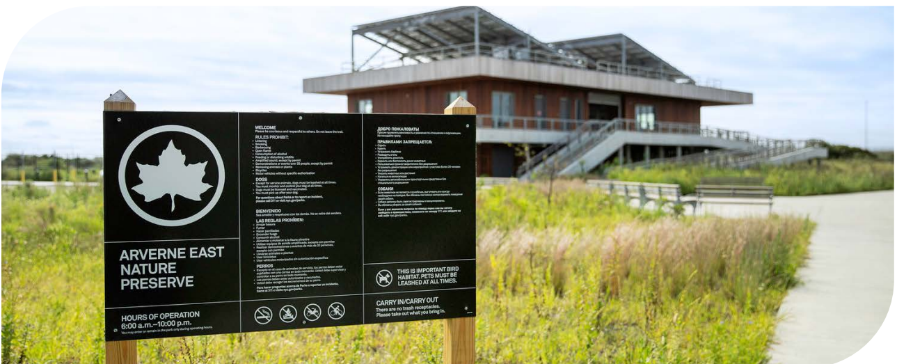
Arverne East will be the first net-zero community in New York City. It will transform a once vacant waterfront site into mixed-use development that fosters economic diversity while bolstering climate resiliency and energy efficiency.
