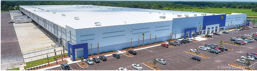
**Best Buy Distribution Center** is a 650,808-square-foot facility that was developed to meet this retailer's surge in online sales. VHB developed an aggressive stormwater approach to significantly reduce fill across the site, which eliminated more than 200,000 cubic yards of import. The result was cost savings of more than \$2 million.
