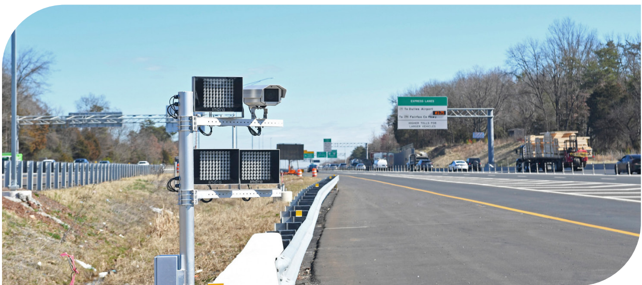
On Virginia's I-66 Managed Lanes, ITS infrastructure provides the real time information agencies need to monitor conditions, manage traffic proactively, and support safer, more reliable travel.
