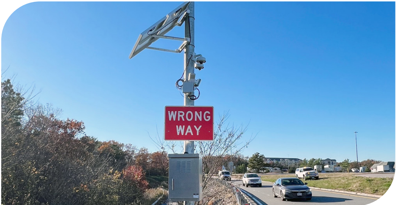
Wrong-way driving detection systems combine ITS technology, real-time monitoring, and operational response strategies to help agencies identify potential threats, communicate critical information, and improve roadway safety.
