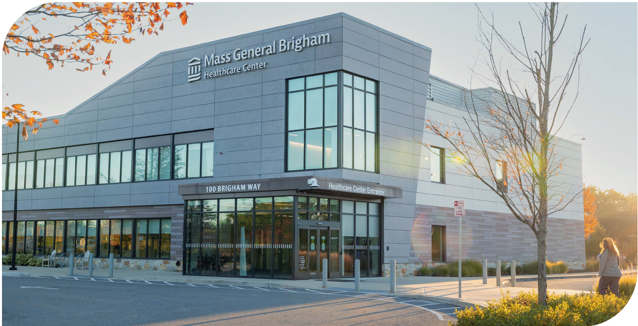
VHB designed the site and utility infrastructure for Mass General Brigham Urgent Care in Westwood, Massachusetts, a suburb outside of Boston.
